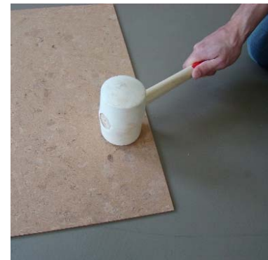
7. Install cork tiles by using a rubber mallet to ensure a proper bond between the two adhesive layers.
