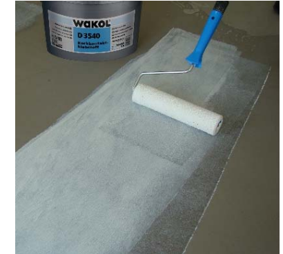
4. Apply adhesive with short-nap roller on the subfloor.
