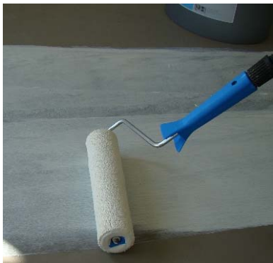
5. Apply a thin layer of adhesive to the subfloor. Ensure full coverage but avoid adhesive puddles.
