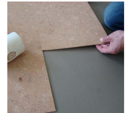
8. Install further cork tiles by using a rubber mallet.
