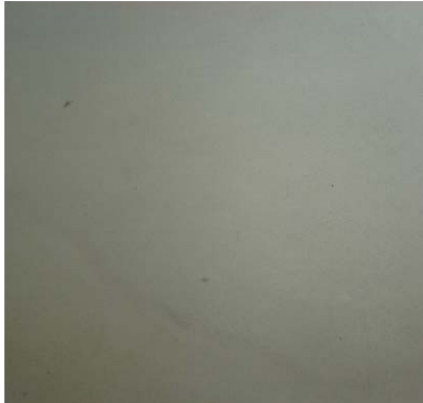
1. Start with a smooth level and dust free cement based subfloor.
